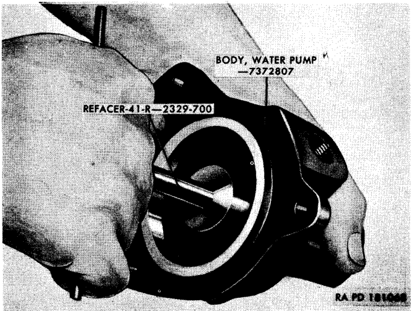
Figure 57. Refacing water pump body seal surface using refacer 41-R-2329-700.
